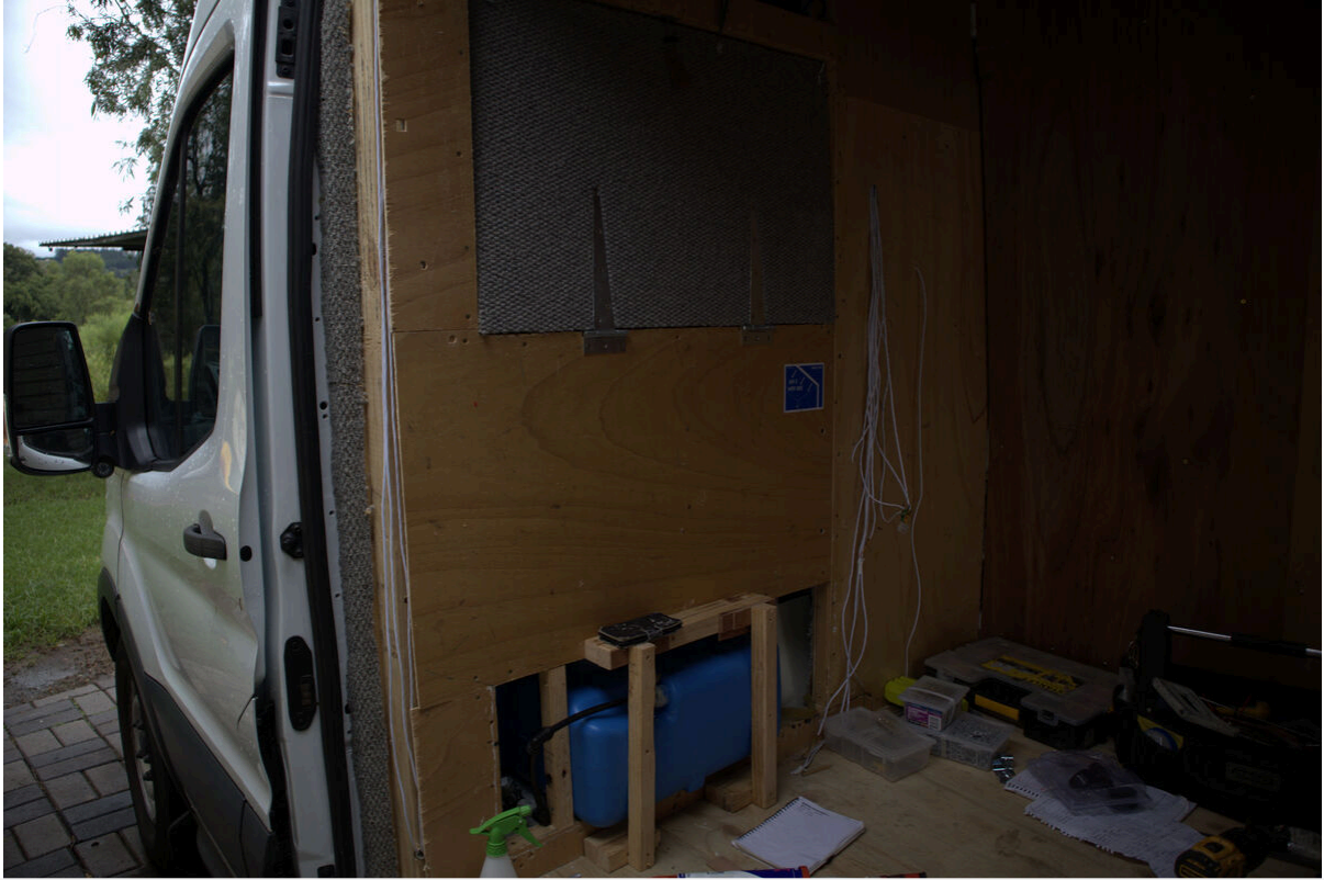
Bare cockpit wall ready for finishing
