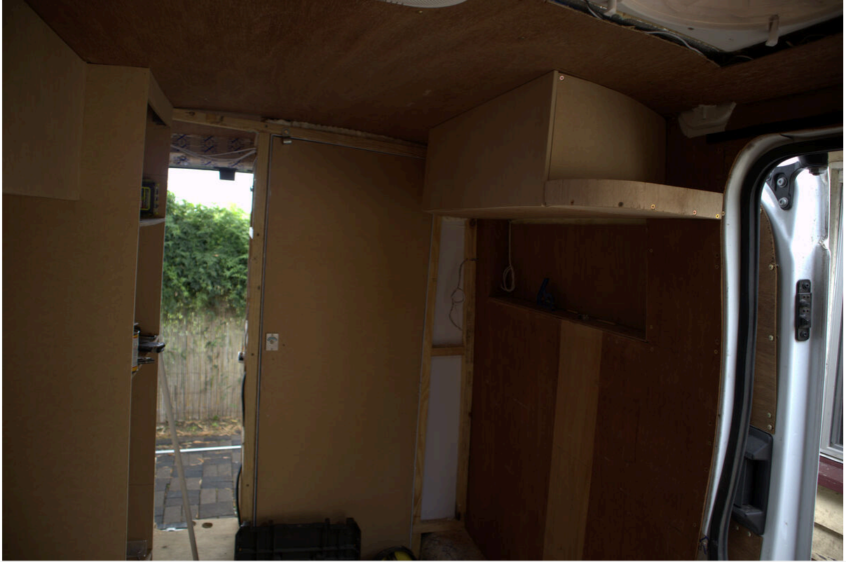
Kitchen area taking shape — bare wood before paint
