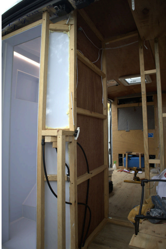
Pipe runs to the shower area before everything was sealed up
