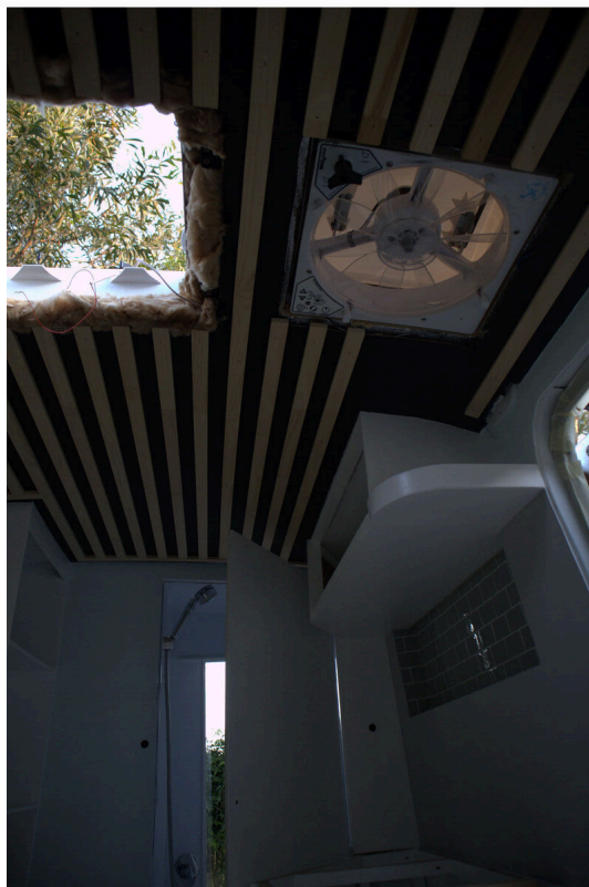
Pine strips going onto the black-painted roof — creating that modern finish
