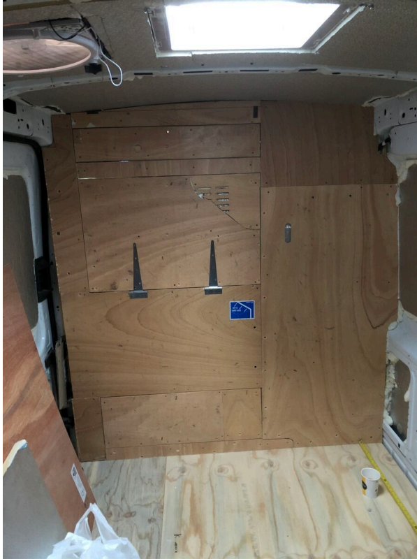
Completed dividing wall with hatch window
