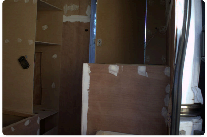
Before and after wood filling — every screw hole and gap smoothed out
