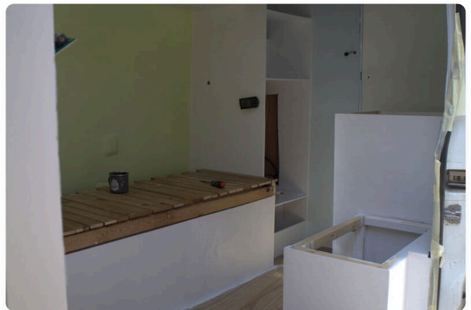
Freshly painted — primer, undercoat, then final finish
